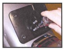
Mount the new bracket assembly using the hardware and rubber gasket provided.
